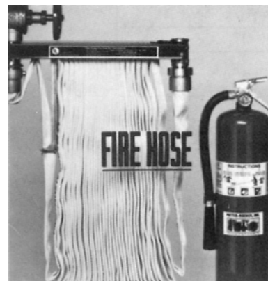
FIGURE A.3.3.19.4 Semiautomatic Hose Rack Assembly.
